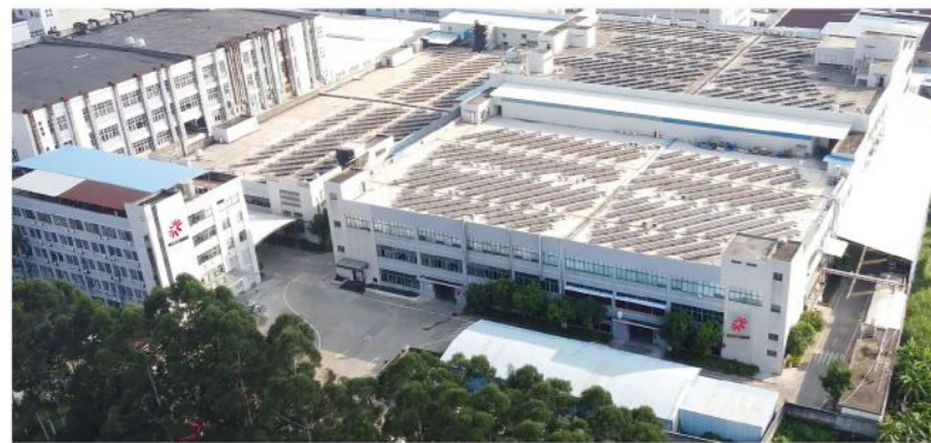
Amitime Manufacturing Center in Zhongshan, Guangdong
